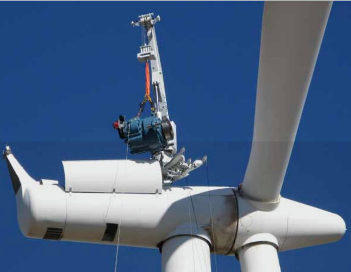
Lifting a piece of machinery from one location to another can be a challenge, particularly when it weighs several tons. Imagine exchanging major wind turbine components weighing more than 20 tons on a wind turbine 100 metres above ground level. This is Liftra's daily challenge.
